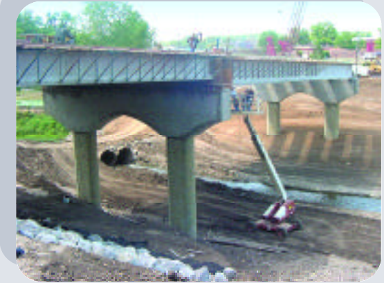
LYDIA BRIDGE OVER INDIAN CREEK
