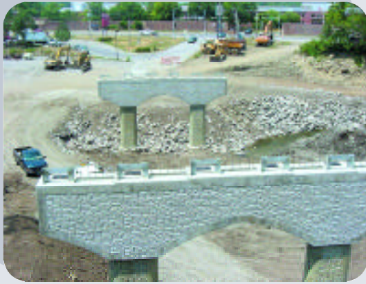
LYDIA BRIDGE OVER INDIAN CREEK
