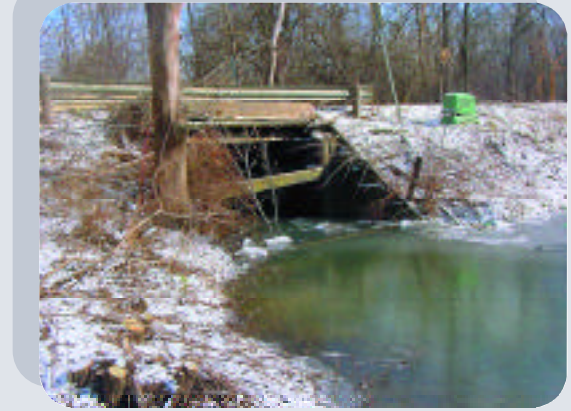
CULVERT AT 155TH AND LUMKINS FORK
